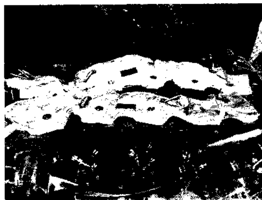
Damaged insulation around burners.
